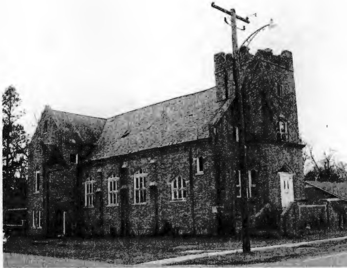
The 1920 Presbyterian Church at the southwest corner of Main and Elm Streets, photographed by Thomason and Associates in 2008, is of the Gothic Revival style.
