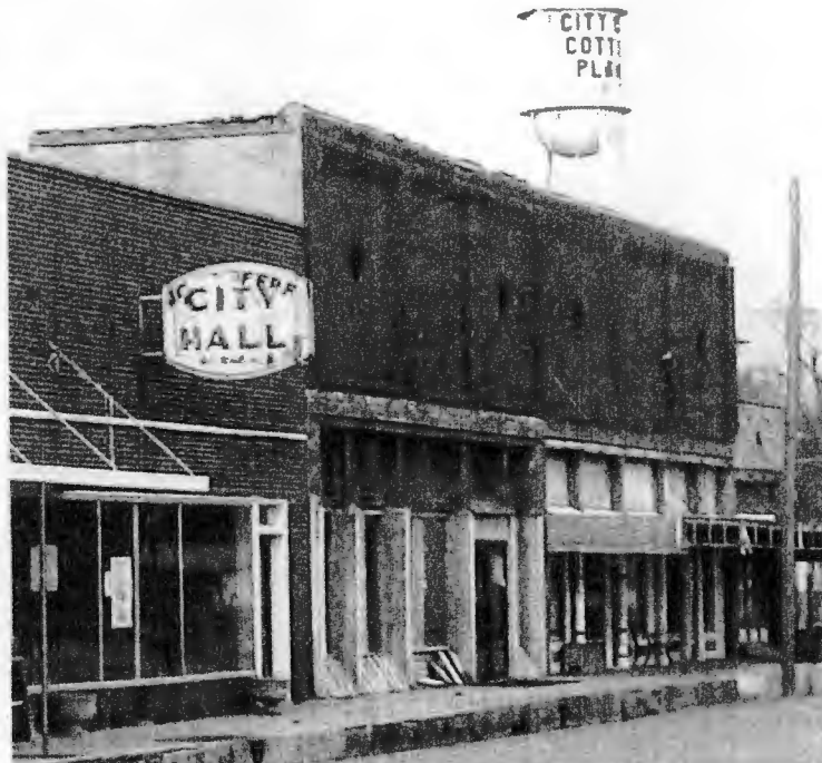
The Leader Company store was located in this two-part commercial block building, a design typical of small town business districts of the early-20 th century. Above the display windows and entrance were transom lights, sometimes with an awning. Below the cornice of this example is decorative brick corbelling. Thomason and Associates photographed the building in 2008.
