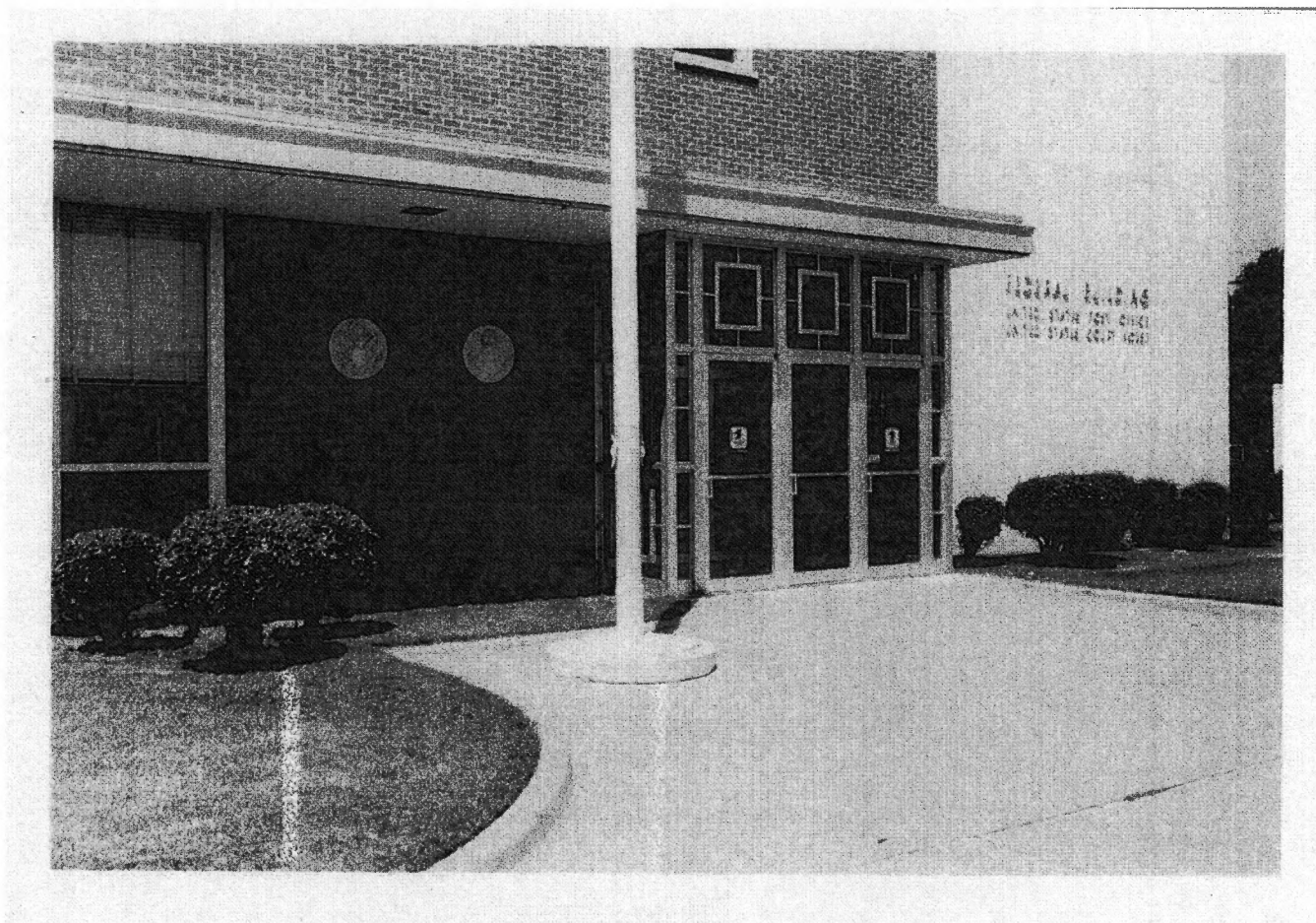
View of main entry, U.S. Post Office and Courthouse, Helena, Arkansas (GSA EDOCs Photo 3958; unknown date).
