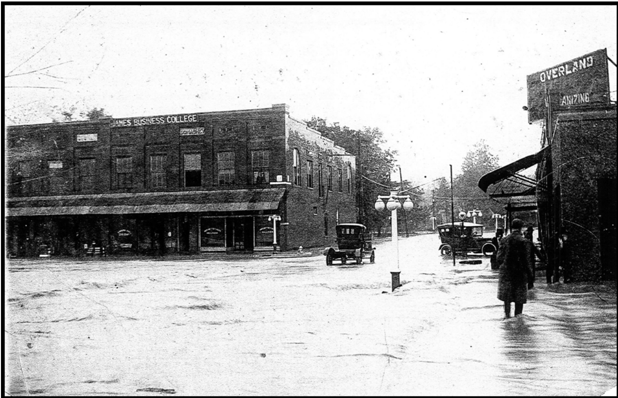
Figure 6. Photograph of Parkway (formerly Railroad Avenue) and Oak streets from the April 1927 flood in Conway, viewing south-southwest. The Donaghey Building (FA0700) is on the left side of the photograph. [Courtesy of the Faulkner County Historical Society Photograph Collection at the University of Central Arkansas.]
