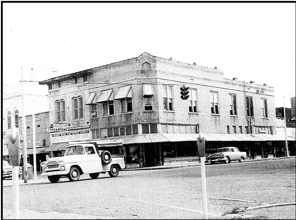
Figure 10. ca. 1958 Photograph of Front and Oak Street intersection, viewing north. The ca. 1960 McNutt Building (FA1075) is now located at the corner of this intersection but the left side of the 1879 Max Frauenthal Building (FA0645) is still extant. [Courtesy of the Faulkner County Historical Society Photograph Collection at the University of Central Arkansas.]
