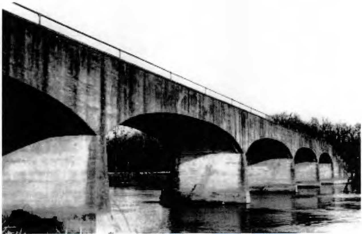
Spring River Bridge, looking east, March 1939.
