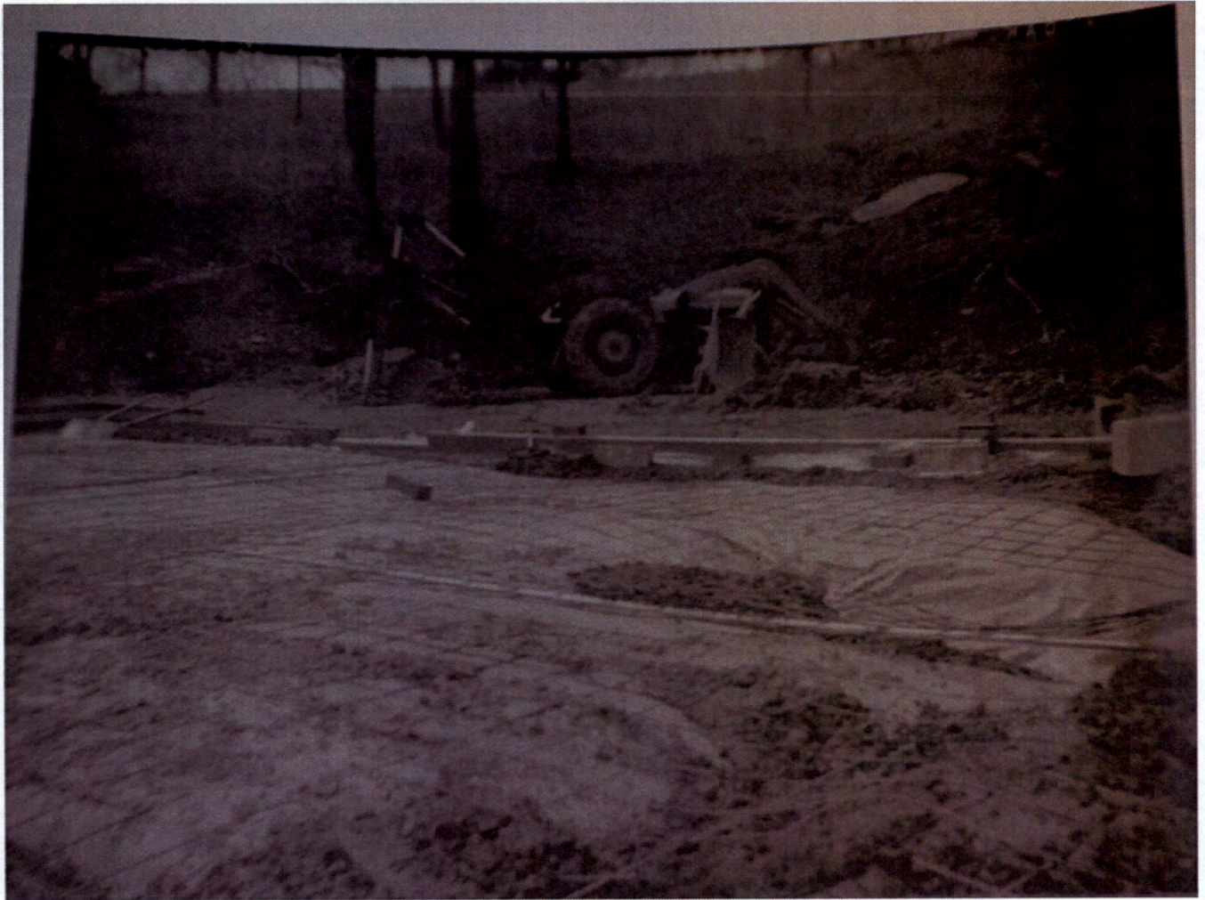
Figure 5: Historic photograph of the Cole House under construction, looking southwest, c.1961. Courtesy of the current owner.
