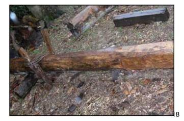
3. Large notches would be made at the end of the logs so the logs would fit together, just like the notches found on Lincoln Logs.
