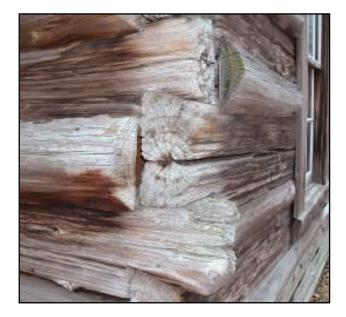
5. Cracks between the logs were filled in.
