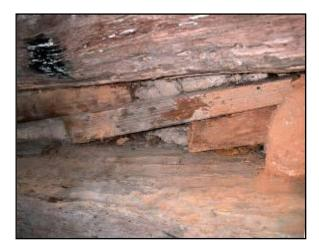
6. The plaster was made of clay or mud, and animal hair was often mixed in to make the plaster thicker. Chinking or daub could be removed during summer for cooling, but added back during winter.
