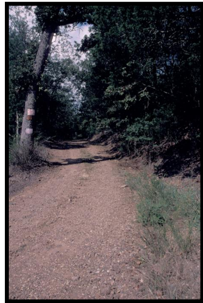
The Cadron Segment of the Military Road, Faulkner County, Arkansas.
