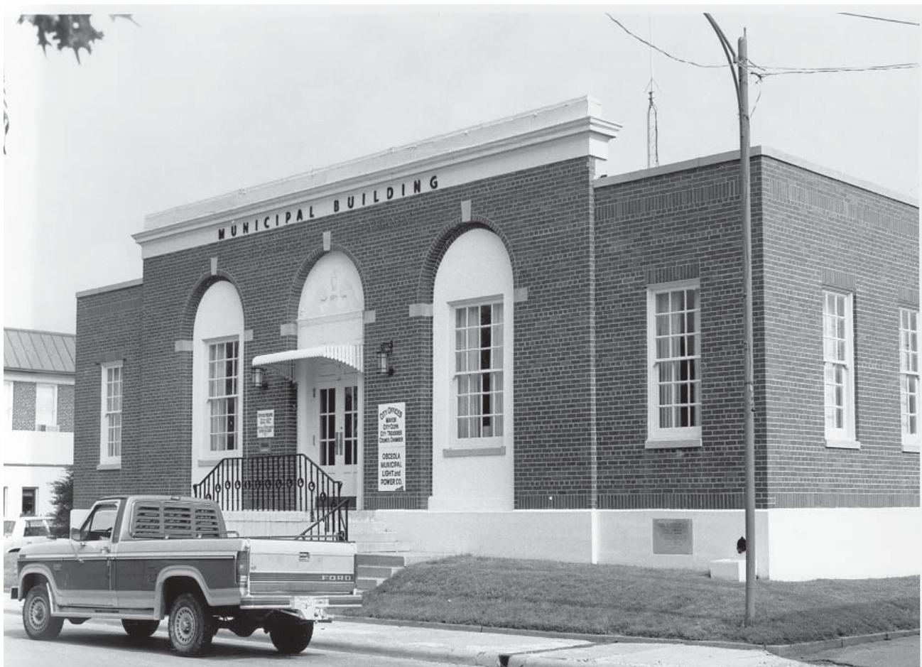
The Osceola Post Office in Mississippi County, built during the Great Depression, held a mural that was later destroyed by fire. (AHPP Photo)
