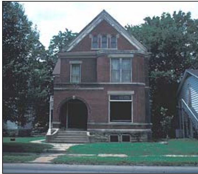
Figure 14: James K. Barnes House, Fort Smith, Sebastian County (c.1893)
