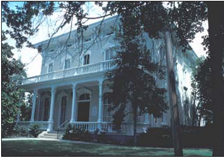
Figure 10: Bonneville House, Fort Smith, Sebastian County (c.1870)
