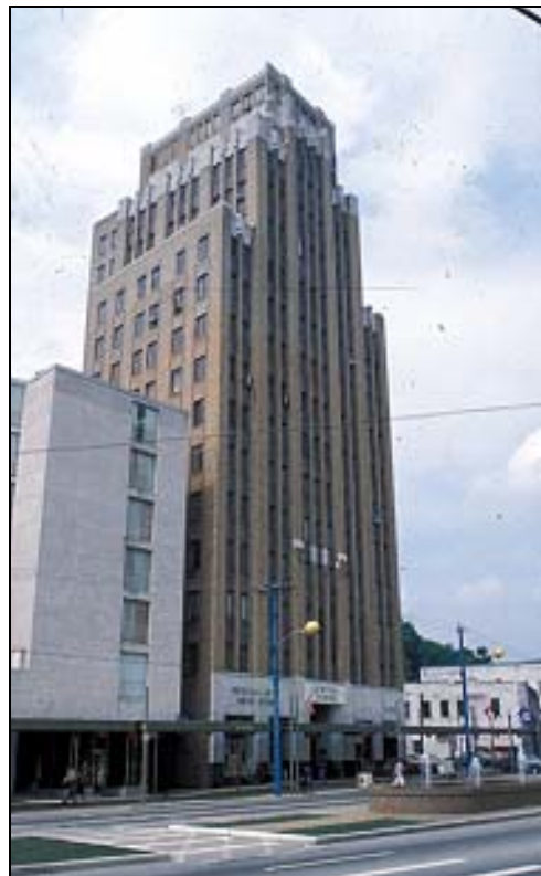
Figure 35: Medical Arts Building, Hot Springs, Garland County (1929)
