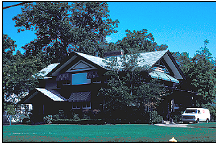
Figure 22: MacMillan House, Pine Bluff, Jefferson County (c.1903)
