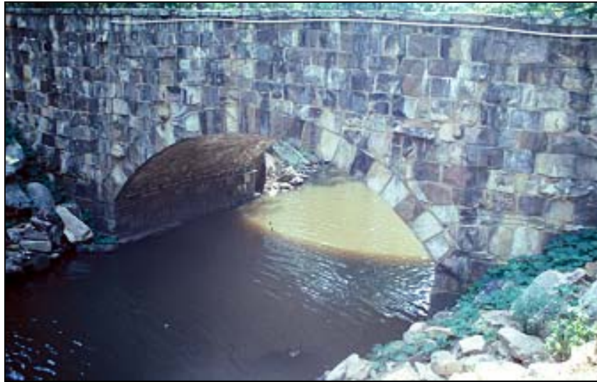
Figure 53: Cedar Creek Bridge, Petit Jean State Park, Conway County (1934)
