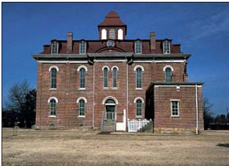
Figure 13: Old Jackson County Courthouse, Jacksonport, Jackson County (1869-1872)
