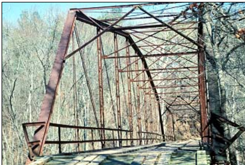
Figure 51: Little Missouri River Bridge, Prescott vic., Clark County (c.1910)
