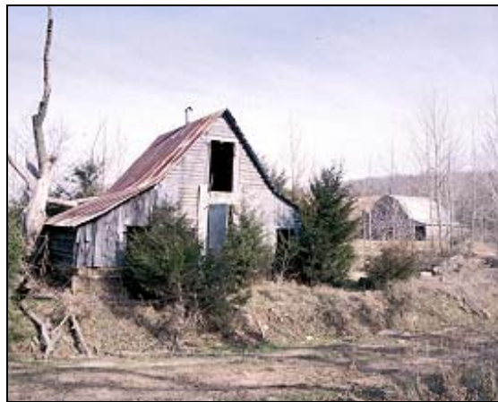
Figure 54: Newton Sutterfield Farm outbuildings, Alco vic., Stone County (twentieth-century)
