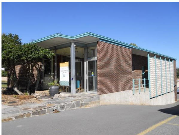
Stowers Building, looking northwest
