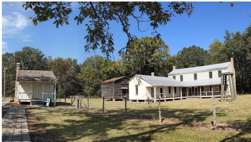
The Taylor Log House after restoration, including the attached kitchen ell, the smoke house, and enslaved quarters.
