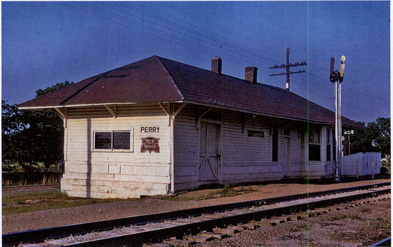
Figure 3: Perry Depot, looking northeast, May 1967.
