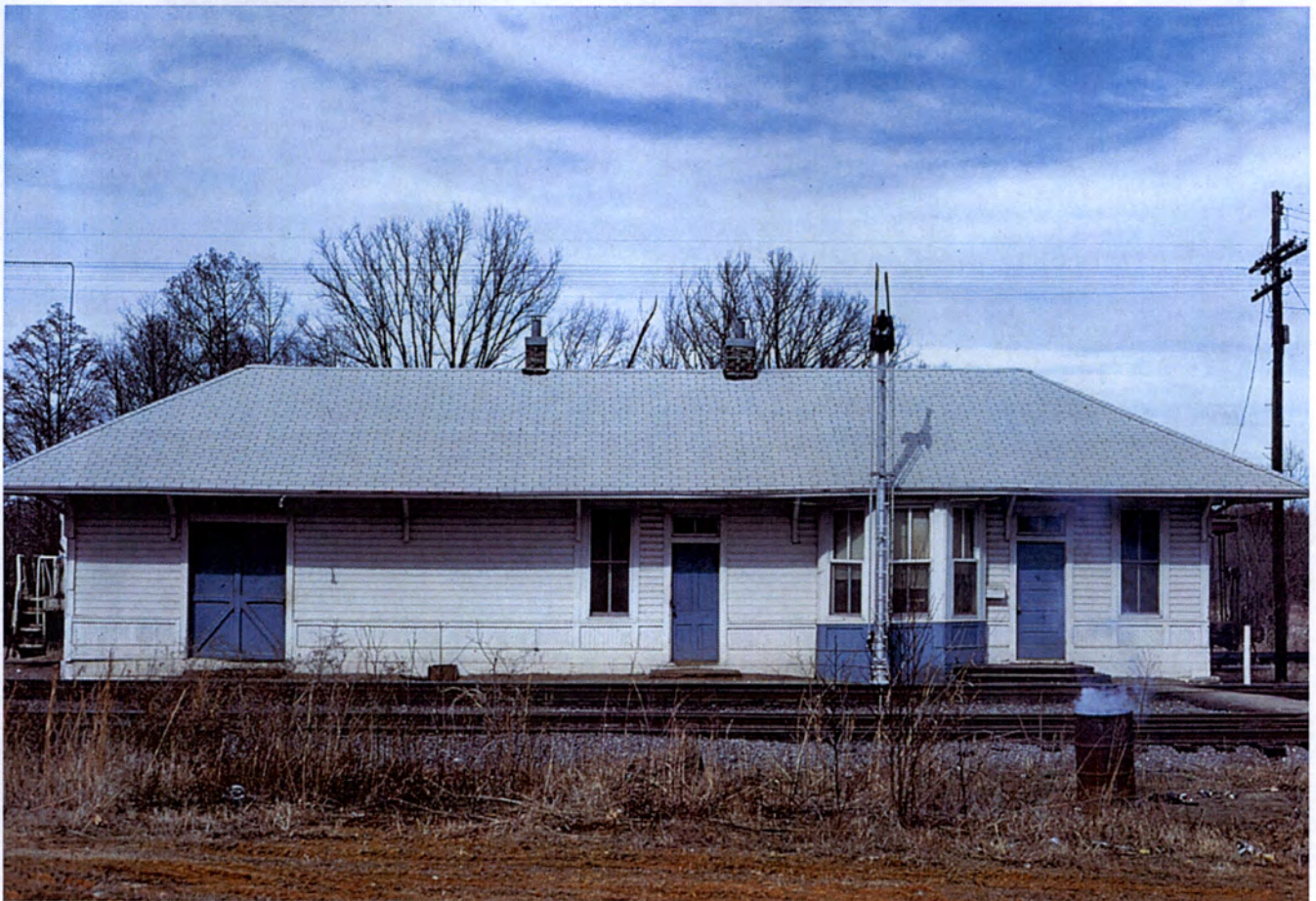
Figure 2: Perry Depot, looking north, February 1980.
