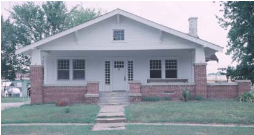
Hunter-Coulter House, Ashdown, Little River County. AHPP Photo.
