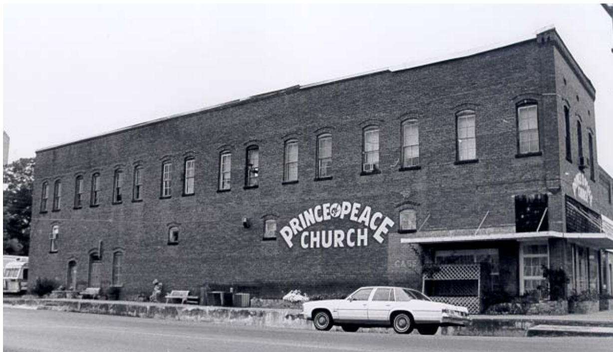
Anderson-Hobson Mercantile Store, Foreman, Little River County. AHPP Photo.
