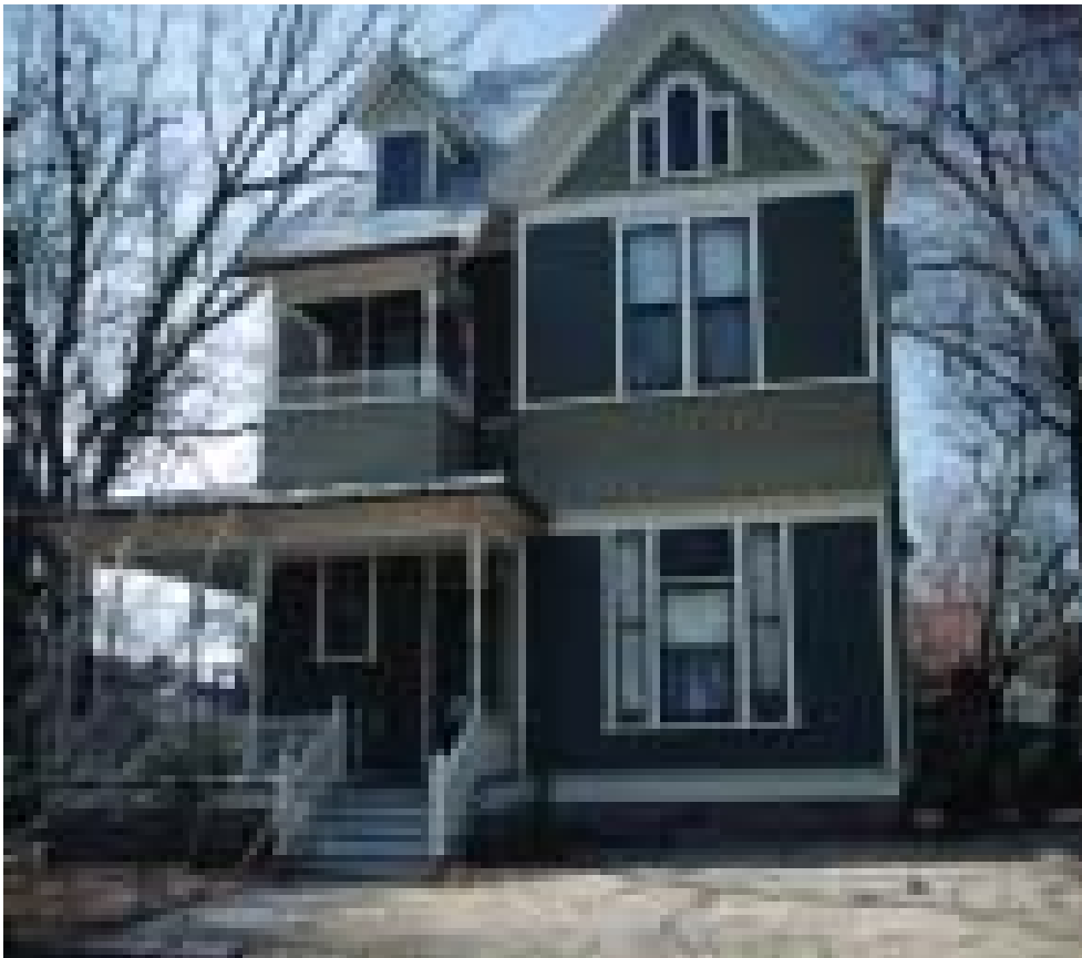
The Martin A. Sharp House at 1422 Summit St. reflects the Queen Anne style of architecture. (AHPP Photo)
