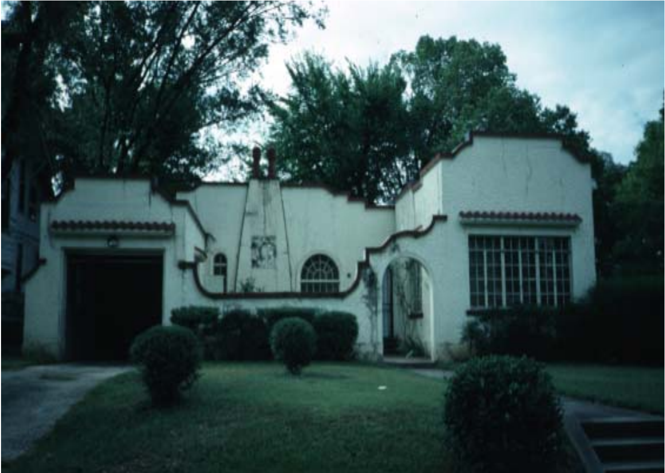
This small house at 1919 West 21st St. is an excellent example of Spanish Revival architecture. (AHPP Photo)
