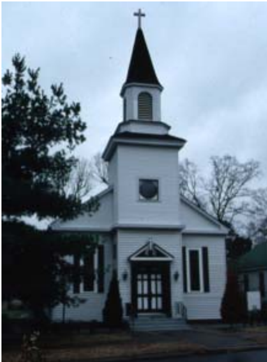
Saint Bartholomew’s Catholic Church, 1622 Marshall St. (AHPP Photo)
