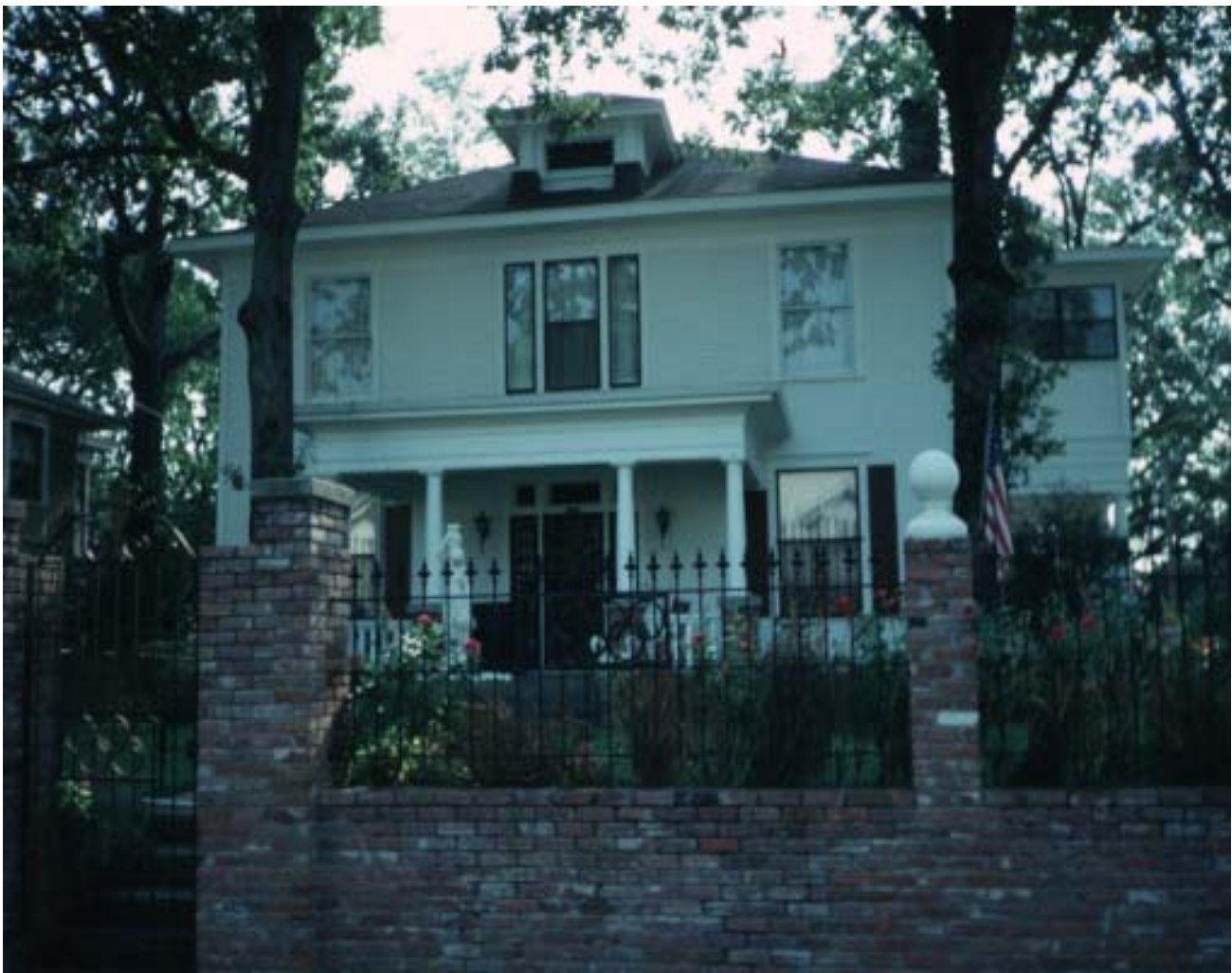
The ca. 1913 Pugh House at 2323 Battery St. is an American Foursquare house with Prairie-style influences. (AHPP Photo)
