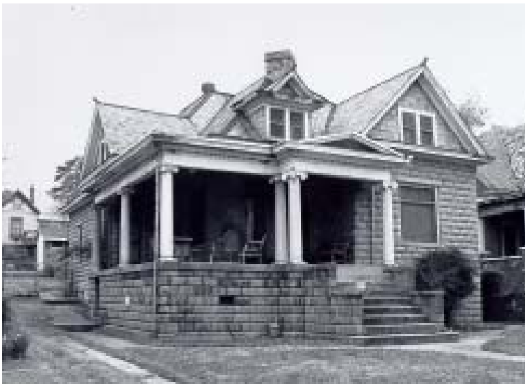
The T.R. McGuire House at 114 S. Rice is a spectacular treatment of the Colonial Revival style of architecture. AHPP photo.
