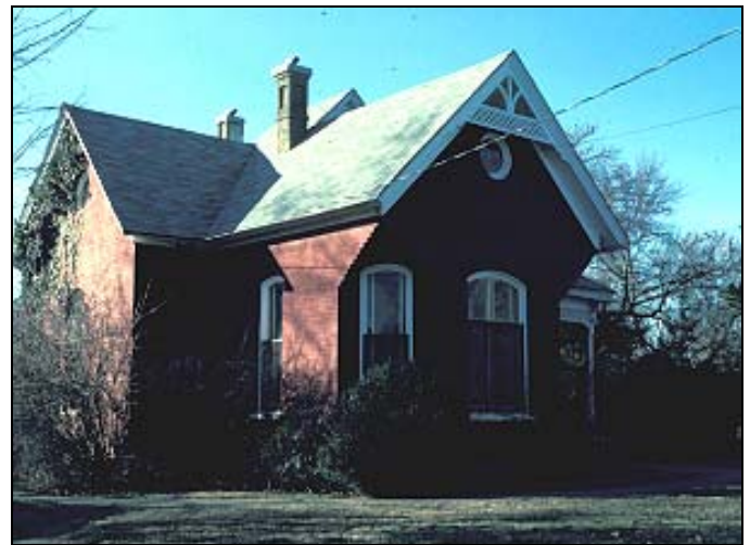
Figure 17: Vinson House, Rogers, Benton County (c.1900)
