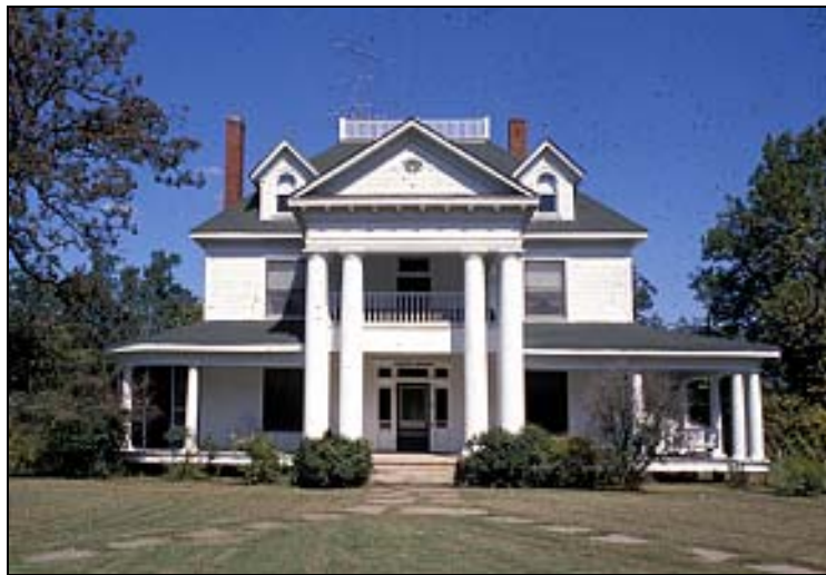
Figure 20: Galloway House, Clarendon, Monroe County (1910)
