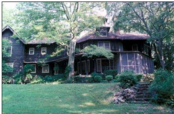
Figure 27: Fordyce-Ricks House, Hot Springs vic., Garland County (c.1909)
