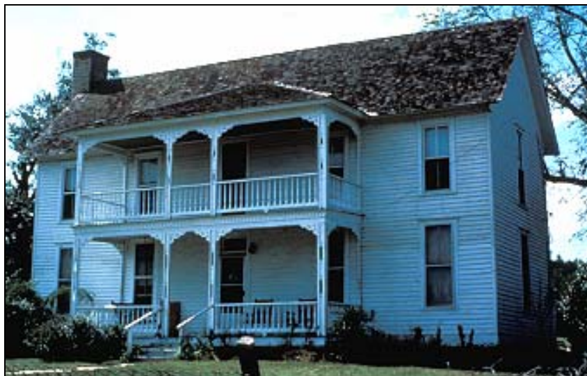
Figure 47: Thomas Hess House (I-House), Marcella, Stone County (1900)
