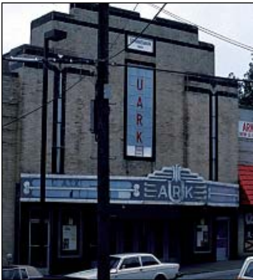
Figure 34: UARK Building, Fayetteville, Washington County (1940)
