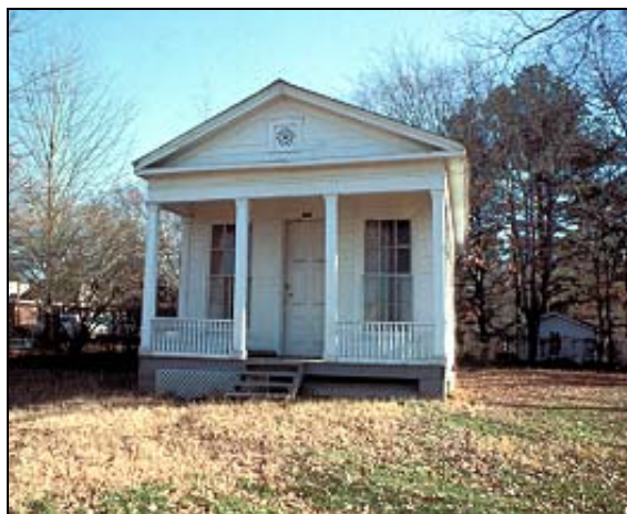
Figure 7: Leake-Ingham Building, Camden, Ouachita County (c.1850)
