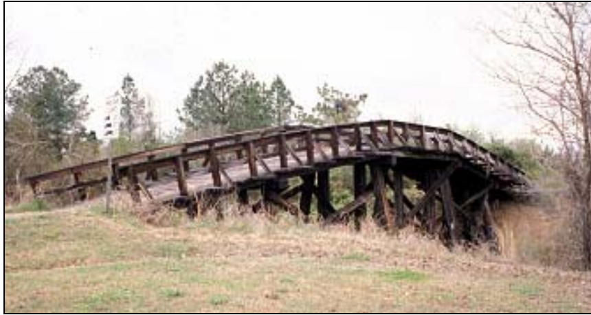
Figure 52: Union Pacific Railroad Overpass, Okolona, Clark County (twentieth-century)
