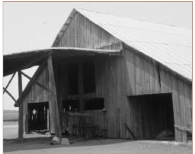
Walls Farm Barn, Tomberlin.
