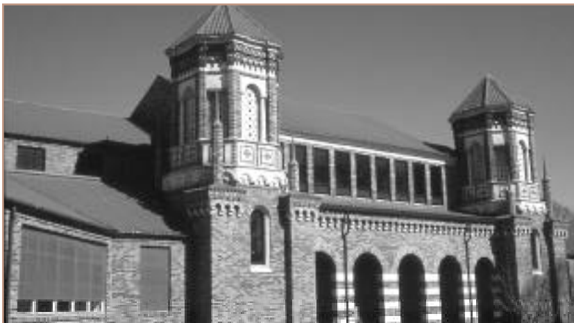
Bentonville High School, Bentonville.
