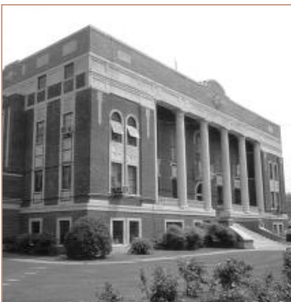
Lonoke County Courthouse, Lonoke.
