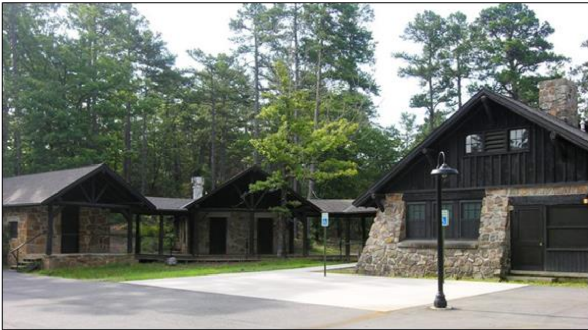
Restored Great Hall (to right) and staff housing at Camp Ouachita
